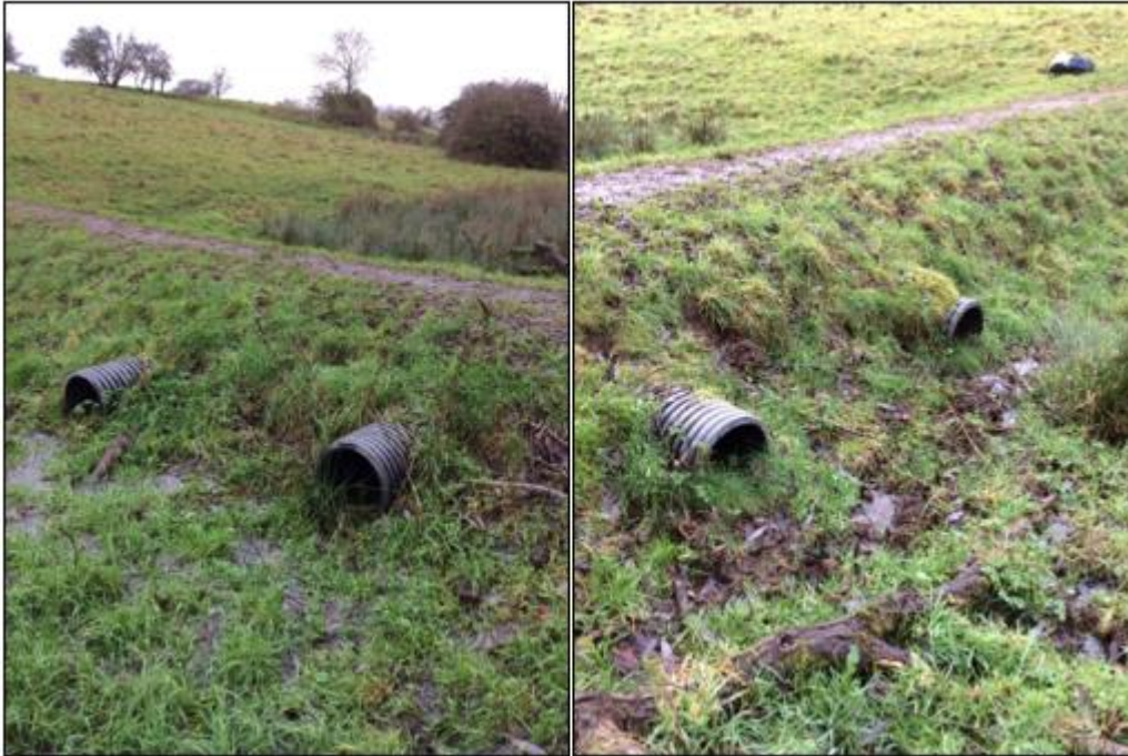
Figure 2-8 Raised and culverted footpath
