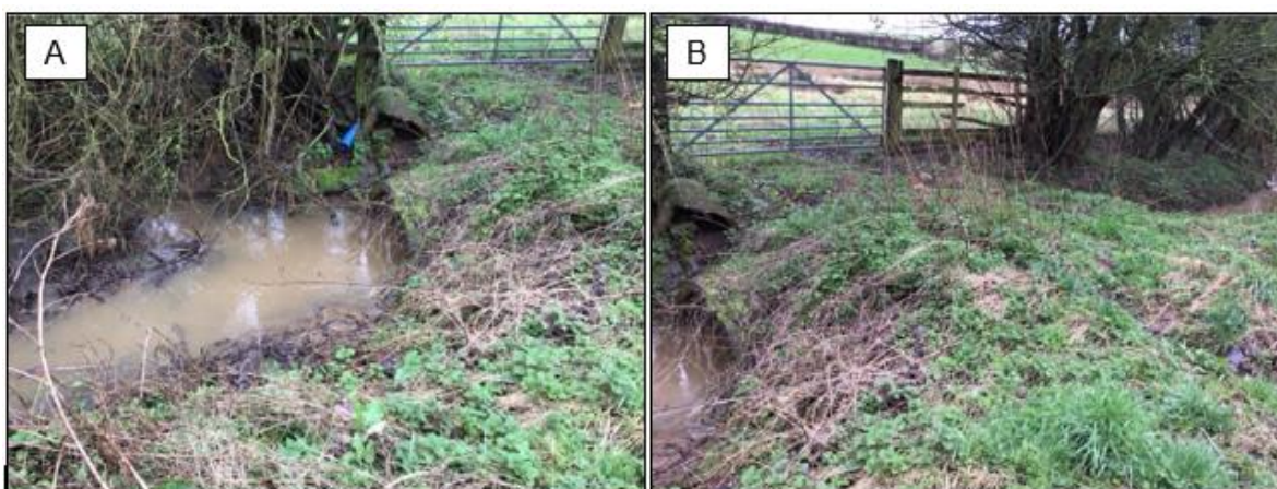
Figure 1-61 On the left bank of a field drain looking at A) the outfall for the field access culvert, B) the entire structure of the field access culvert. In B the field beyond the fence is full of rushes and a potential paleochannel or low relief that is holding water from the flow path seen in Figure 1-61 D
