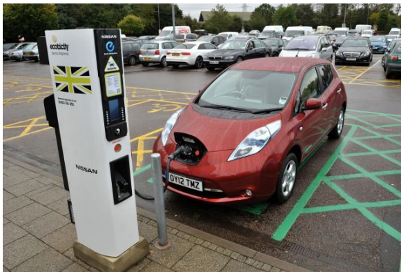
Figure 5: Electric car charging bay
