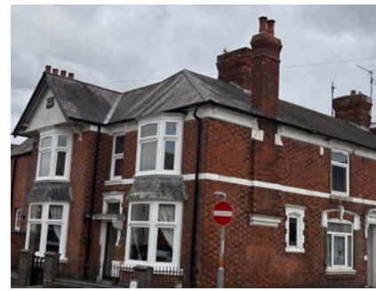
41. Prominent corner building
