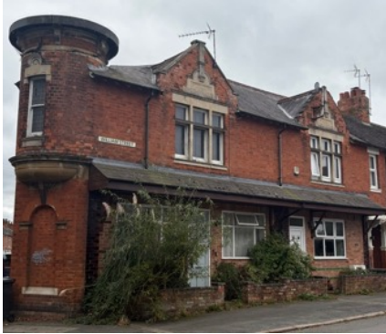
17. Prominent corner building
