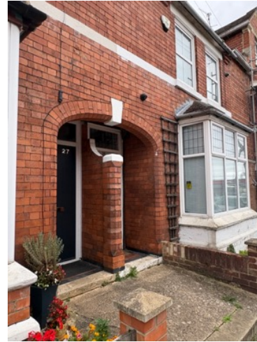
3 Flattened door archway
