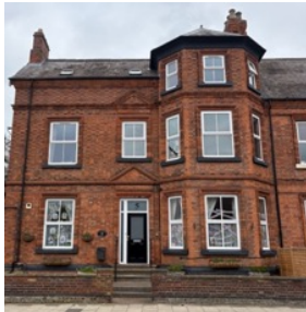
33. Three storey canted bay
