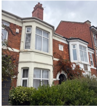
26. Two storey canted bays
