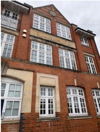
25. Prominent former factory
