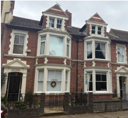
21. Two storey bays plus dormers
