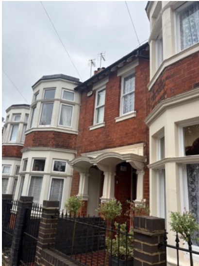
9 Two storey polygonal bays
