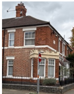
39. Distinctive battlemented parapet
