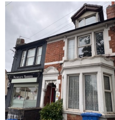
32. Single storey canted bay
