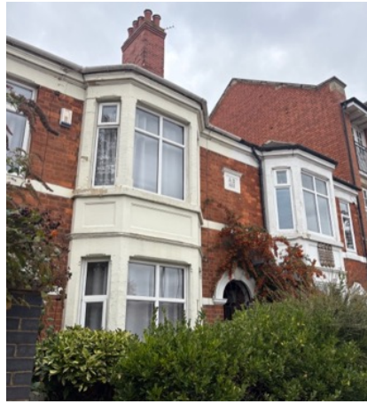
26. Two storey canted bays
