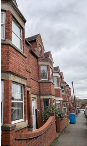
1 Two storey canted bays
