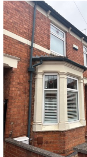
11 Single storey canted bay
